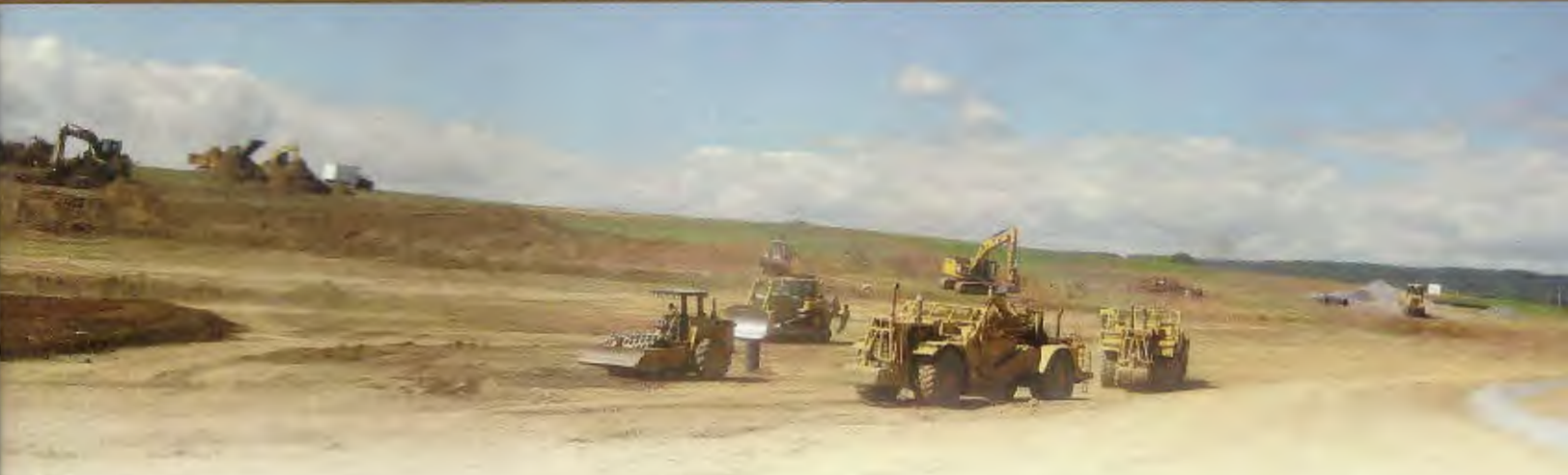
BCBP II Construction
