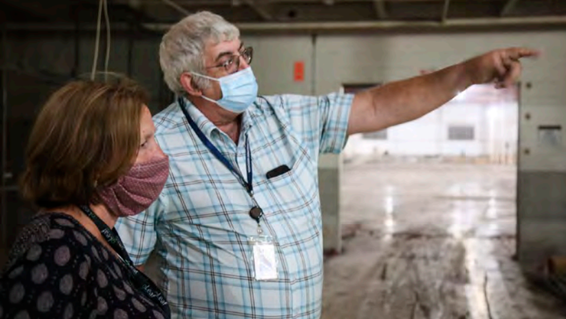
Alan Mountain, Greenleaf, gives Bette Slayton, BCDA, a tour of the facility currently under construction for the $30 million Phase II project
