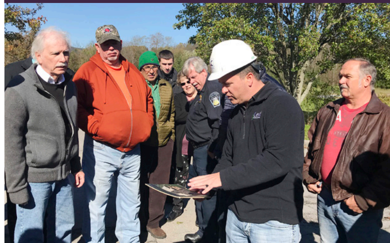
Green Leaf Building Tour: Saxton Mayor Alan Smith, left, and a group of Community Leaders join Phil Goldberg for a tour of the Green Leaf facility currently undergoing a $13 million renovation to house the new medical cannabis grower-processor facility.
